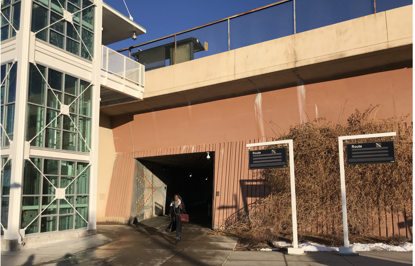
Station access tunnel
