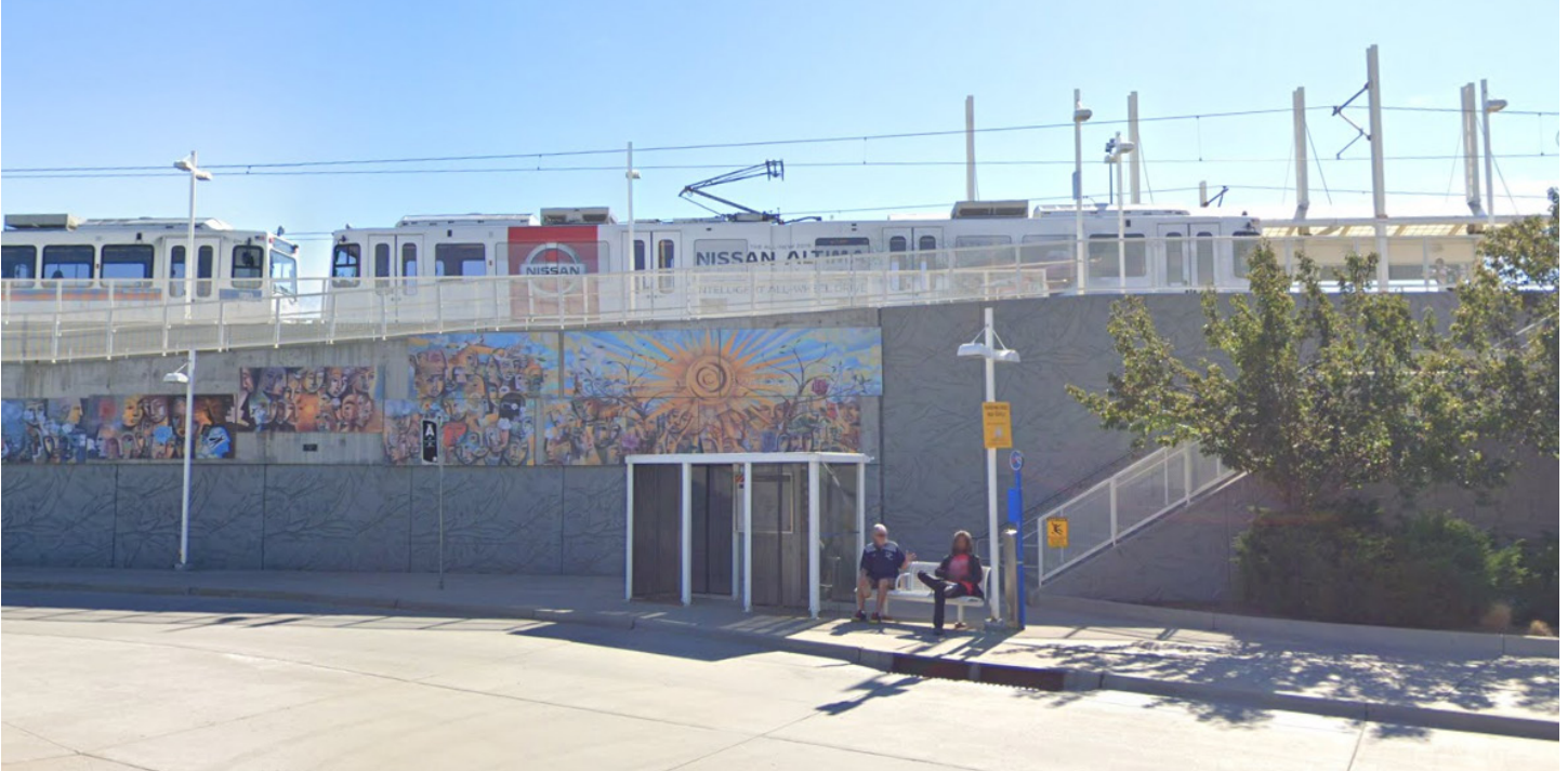
Bus shelter adjacent to station access stairs
