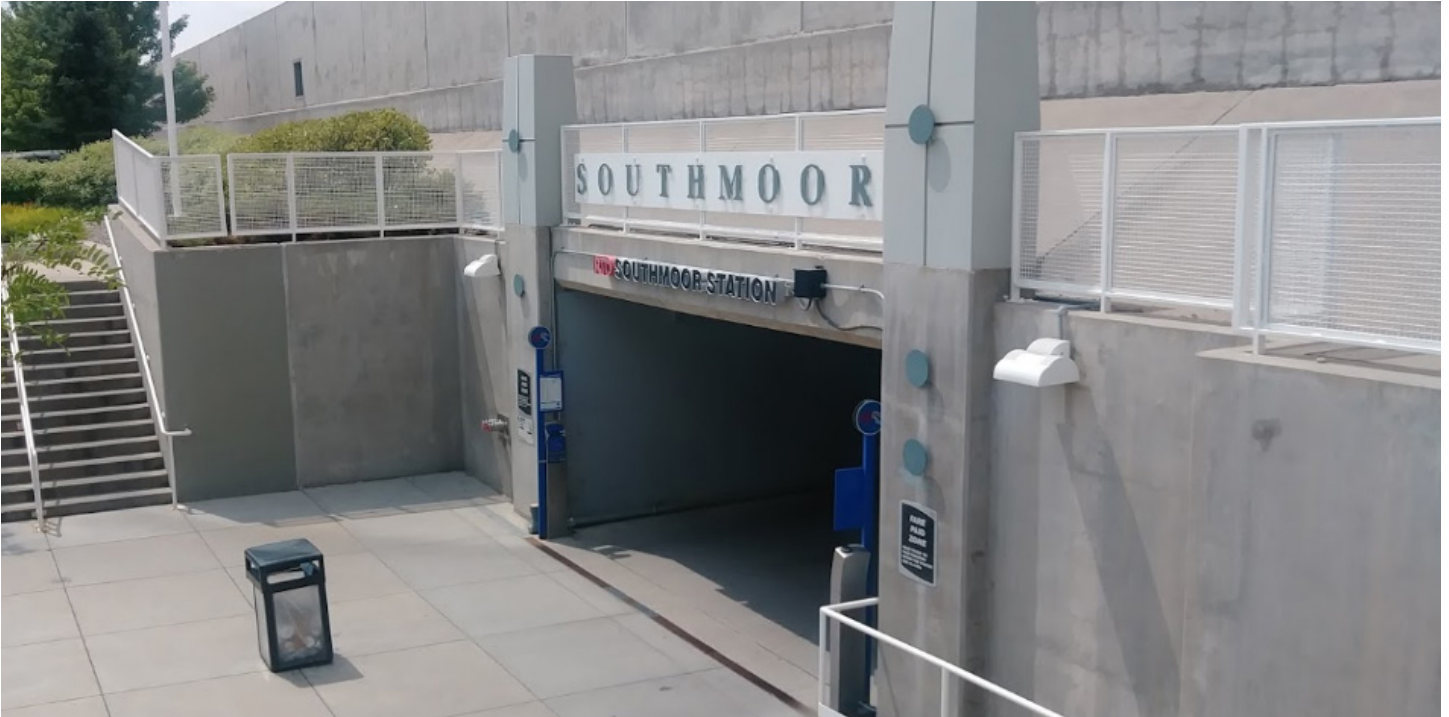
Station access tunnel
